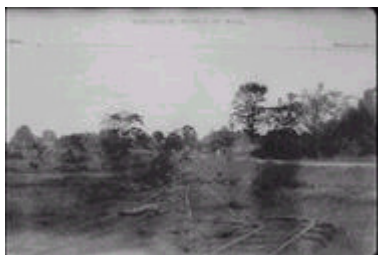
Bent rails at Rangapara, Tezpur-Balipara Tramway
