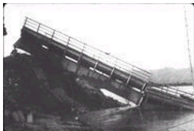
North Lakhimpur, Assam Bridge on Ranganadi Assam.
